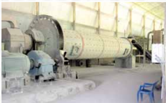
A Cement Manufacturing Unit financed by the Bank
